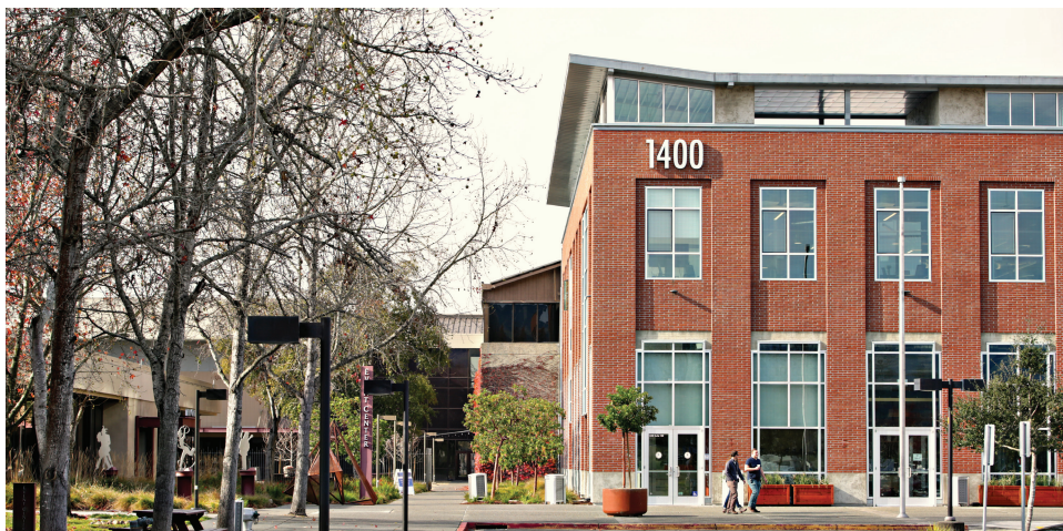
Figure 7. Adaptive Re-use of Building 1 Completed in 2008
